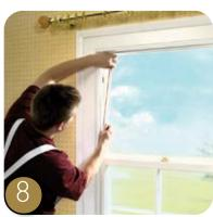
Replace the upper three parting beads - two either side and one spanning the top width of the window [G].
