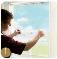
Using one inch masking tape, protect the Weatherfin Pile at the midrail (H) and bottom rail (J) of the bottom sash (F).
