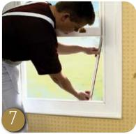
Once painted, remove the masking tape from the staff beads (I), the midrail (H) and bottom rail (J) of the bottom sash and replace the two lower parting beads.
