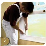
Slide the bottom sash (F) up and ease out the lower two parting beads (C) from either side of the frame.
