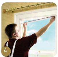
Remove the parting bead (C) that spans the top width of the window.
