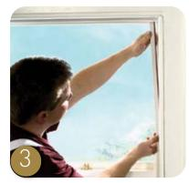
Pull down the top sash [E] remove the two upper parting beads [C] from either side of the frame.
