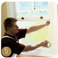
The sashes will now move more freely with the parting beads removed. Using the masking tape, protect the Weatherfin Pile in the staff beads (I).
