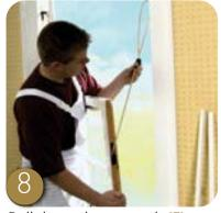
Pull down the top sash (F) inwards and unhook the sash cord holders on the top sash as described in Steps 3 & 4.
