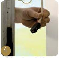
Pull the sash cord holder (I) down and out from the cord housing (J). Repeat steps 3 & 4 on the opposite side.
