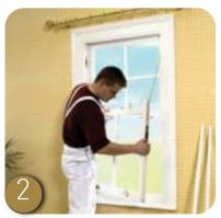
Lift out the bottom sash (G) and rest it internally on the base of the window.
