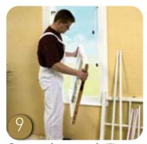
Remove the top sash (F) internally, allowing easy maintenance, cleaning and painting.
