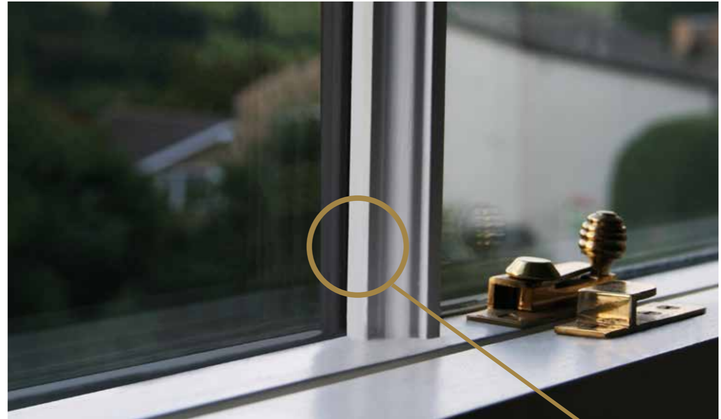
Single Glazed (normal glazing bar)
